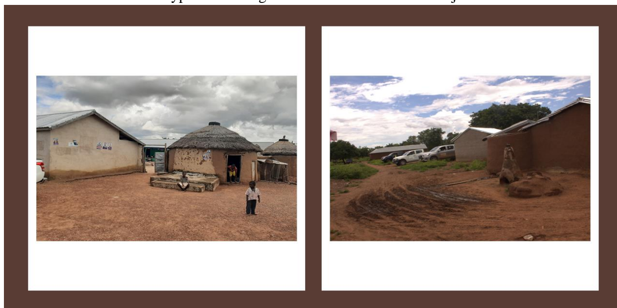
Plate 4-7: Typical Housing Infrastructure Within the Project Enclave
