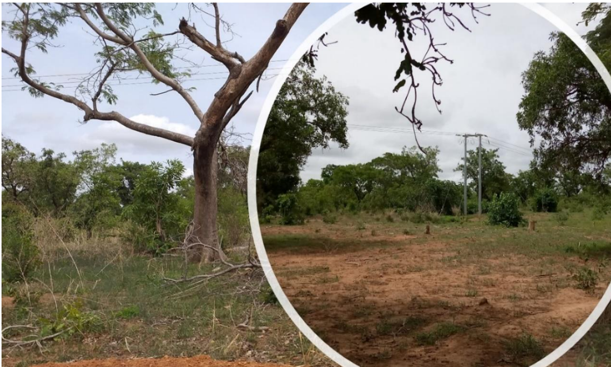
Plate 3-2: Ongoing Development of new 34.5 kV sub-Transmission line by PV Project Site
